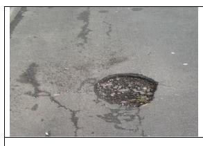
Example of typical pothole in carriageway approximately 250mm diameter, abrupt difference in level, 40mm deep.
